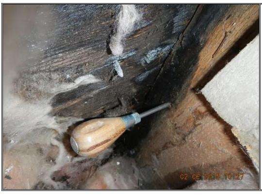
**Description:** Rot damage on stud and wall sheathing
