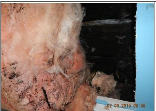
**Description:** Wet insulation and rotted siding
