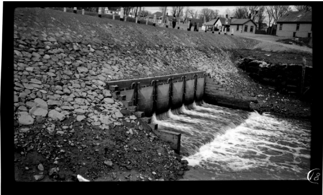
Fresh water flowing out through the clapper valves at low tide, May 9, 1941.
