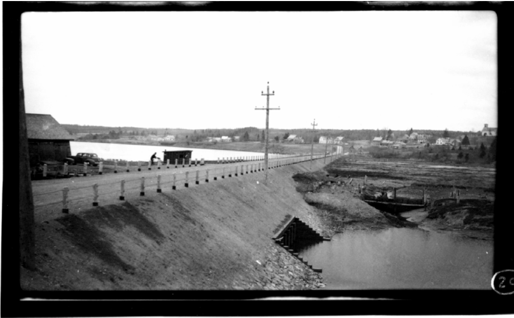
View of the bridge, road, and tide gates in the year following construction, May 9, 1941.
